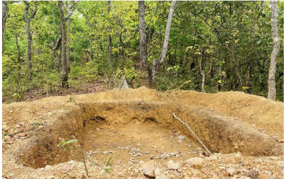
Figure 3 Conservation Pond (Recharge Pit) at Kalika CFUG
