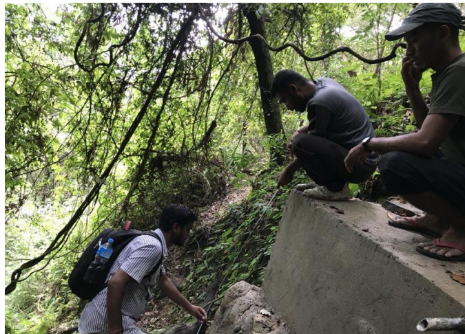
Figure 2 Measurement of water tank supported by project
