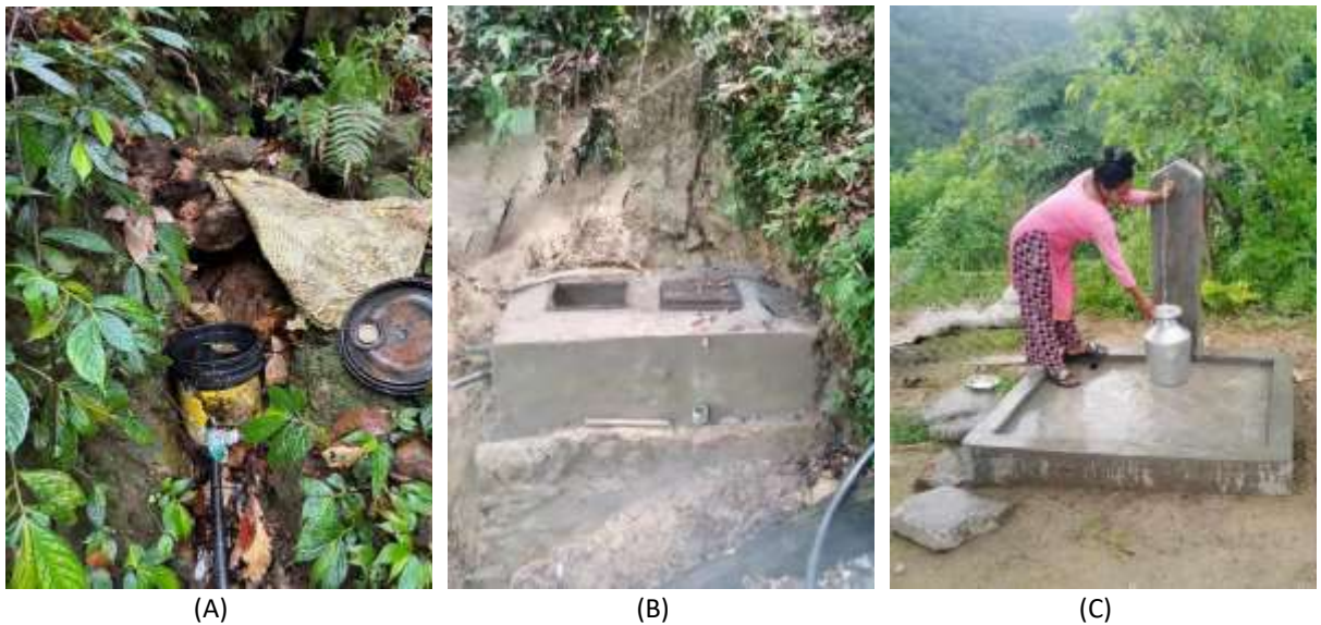
Fig. 2: Restoration and protection of a water source in the Simle sub-watershed, Ghyanglekh Rural Municipality-1, Khattar, Sindhuli
